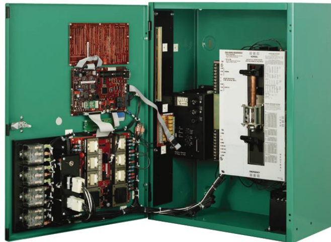
Figure 8. Enclosure Interior of Automatic Transfer Switch.
