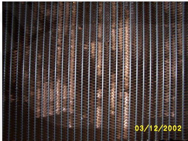
Figure 2-2 Fins damaged by pressure washing at acute angles to core face
