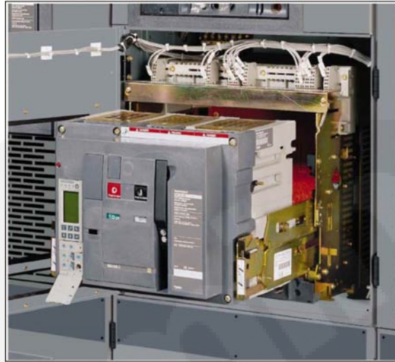
FIGURE 46. INSULATED CASE BREAKER WITH TYPICAL DRAWOUT, SHOWN IN WITHDRAWN POSITION.
